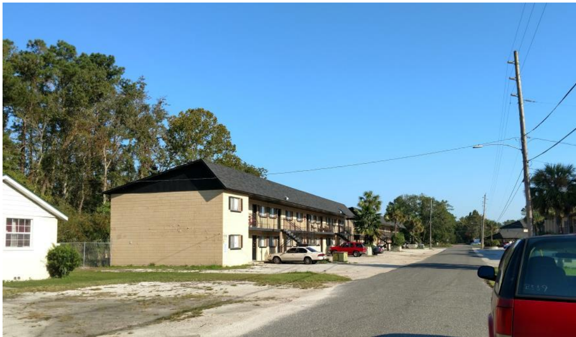
Adjoining property to the west, across Laclede Avenue Source: Staff, Planning and Development Department Date: 09.20.2017
