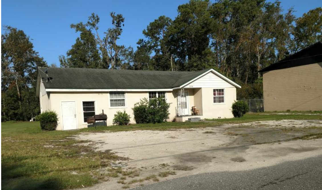
Adjoining property to the west, across Laclede Avenue Source: Staff, Planning and Development Department Date: 09.20.2017
